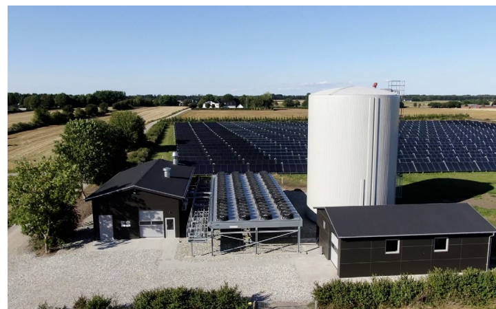
A heat pump can be integrated with other energy sources; e.g. utilized to optimize the efficiency of a solar heating plant
