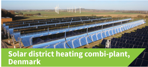
CSP for combined heat&power, Denmark
