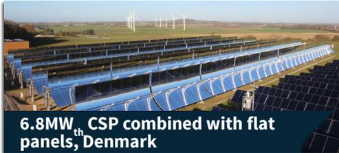
**6.8MW<sub>th</sub> CSP combined with flat panels, Denmark**
