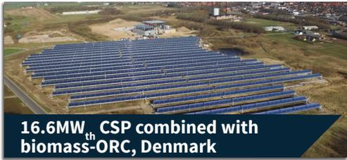
**16.6MW<sub>th</sub> CSP combined with biomass-ORC, Denmark**
